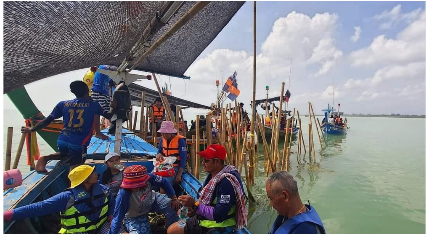
Artificial fish habitat installation
