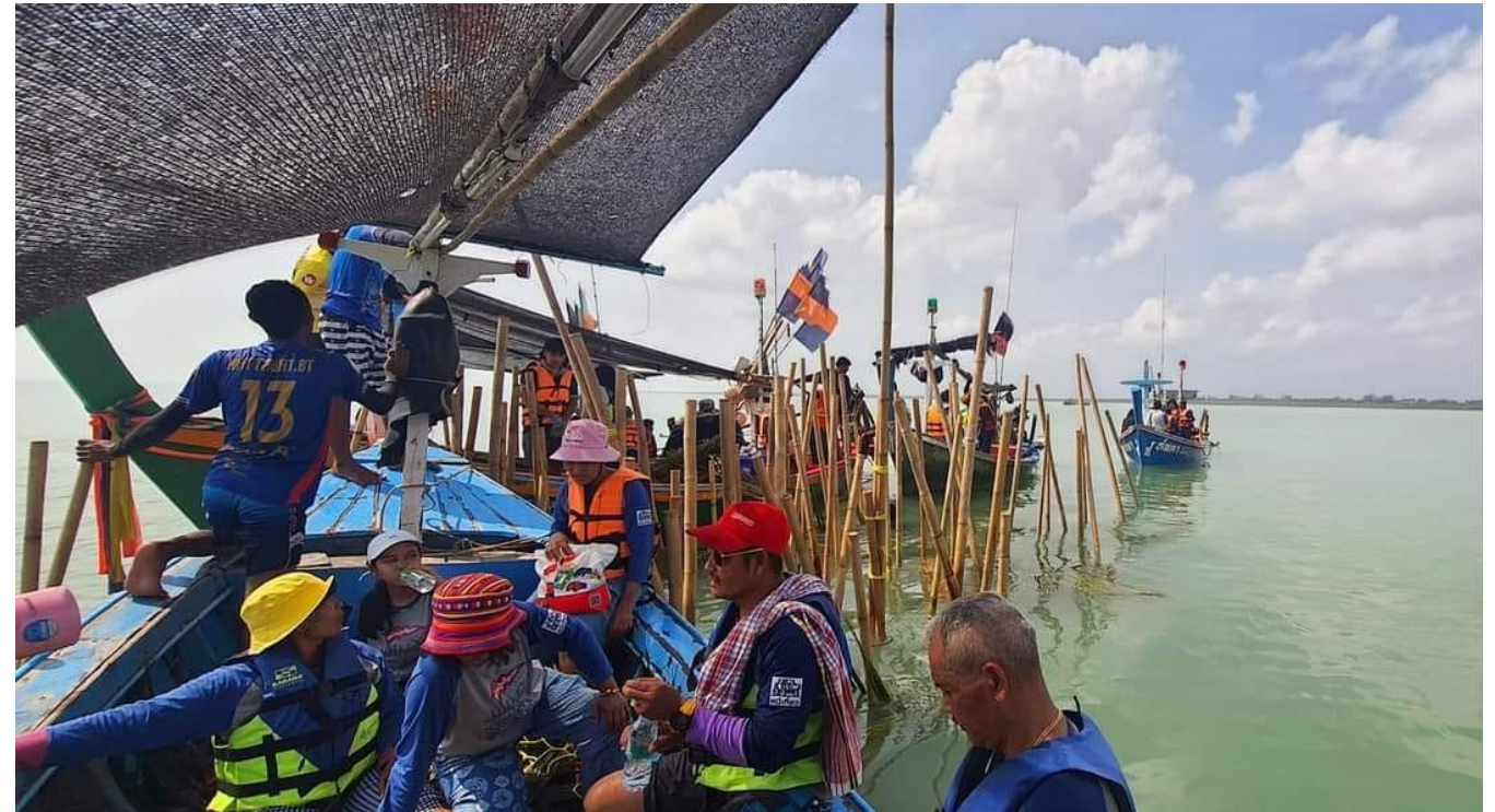
Artificial fish habitat installation
